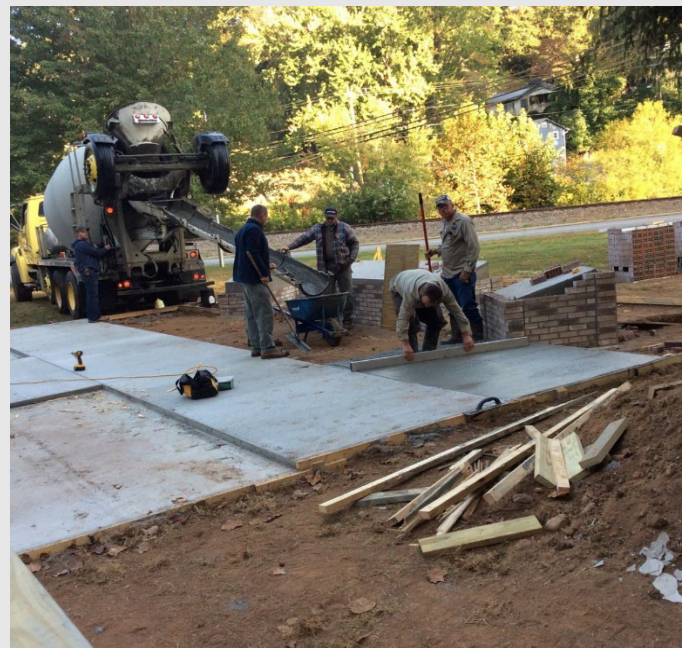
Grounds Crew Working on a Project.
