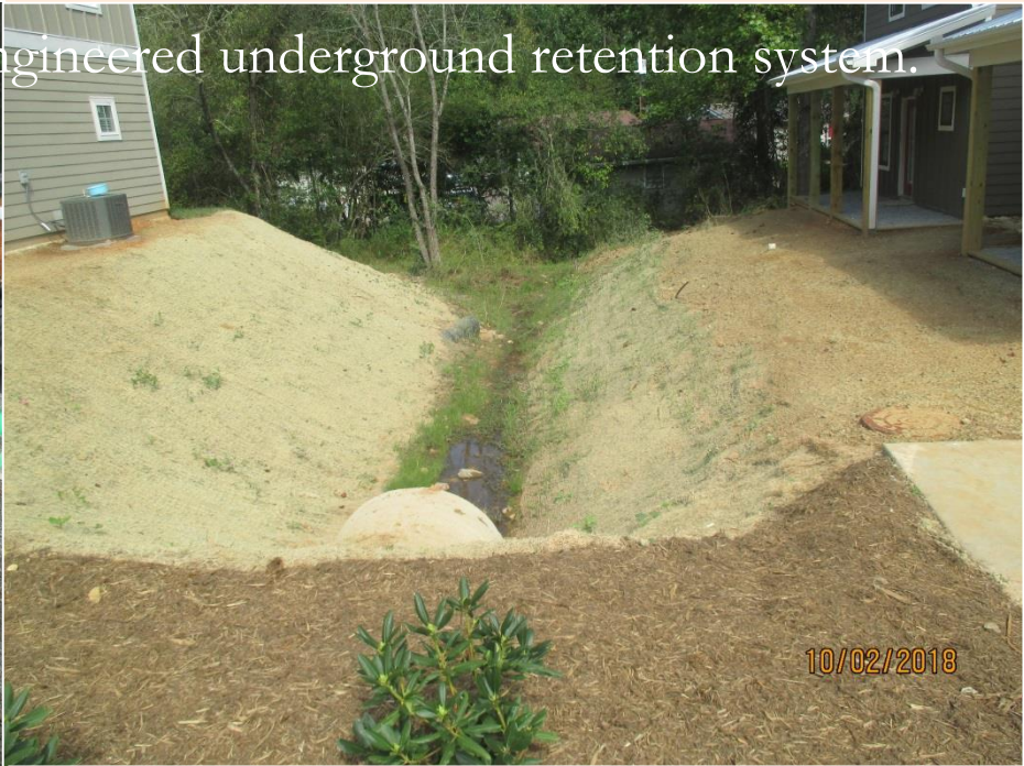
Ditch lines and sediment basins are very important when constructing a new driveway; that water has to run somewhere!
