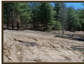
In this photo it is obvious that no attempt to establish ground cover has been made. **Ground cover is the best erosion control measure. Ground cover reduces the need for sediment control. Seed and mulch ASAP. It will rain.**
