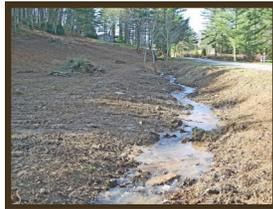
Sites near a stream may require an undisturbed buffer zone. This photo shows a violation of county, state, and federal laws. **Get permission before you dig in the creek. Stream culverts require permission from the Army Corps.**
