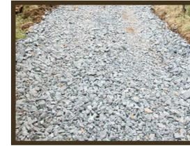
An adequate gravel construction entrance will be 2"-3" clean stone at least 6" deep and 12' wide. **Loose BIG stone scrapes mud off tires.** Small stone will "pack down" and doesn't work as well. **Place stone where vehicles enter the highway.**
