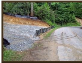
An unsafe condition is created if you allow mud from your site to be tracked onto the public road. **You may be held responsible if it causes an accident.** An adequate gravel construction entrance can prevent a "mud-slick".
