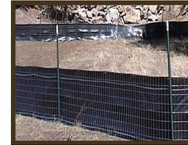
Installing silt fence properly will require the filter fabric to be attached on the **uphill side of the post**. Silt fencing should be buried 4"-6" with **compacted** backfill. Silt fencing is recommended at the toe of the slope and along slope contours.
