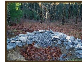
Correctly constructed temporary sediment traps need small stone across the face of the structure a minimum of 1 ft. thick to reduce drainage rate.
