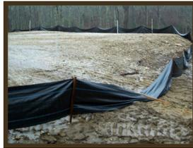
Silt fence that has been installed incorrectly or in an area of concentrated flow will fail. **Silt fence works by reducing water flow and retaining sediment on site.** Silt fencing should be reinforced.
