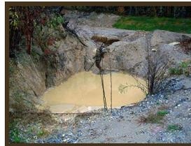
This **temporary** sediment trap needs an outlet spillway section constructed of stone to provide drainage for the pool. The inside face of the outlet section should be lined with gravel to slow the release of drainage water and improve efficiency.
